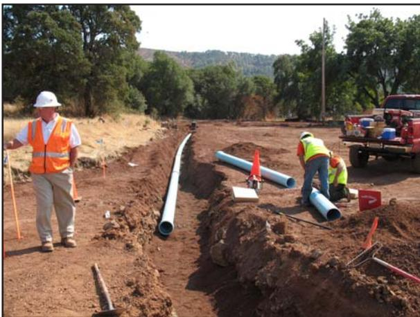
Installation of the new water line
